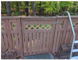
**11:** The gap between the fencing and the decking near the pool pump was too large. Recommend correction for safety.
