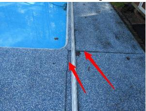
14: The track for the pool cover created a trip hazard around the pool. Cracked as necessary.
