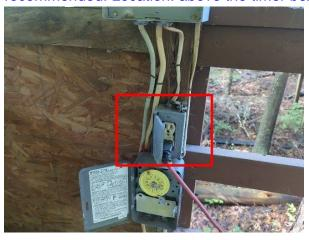
**37:** There was no general purpose receptacle installed in the approved areas around the pool which can lead to the use of extension cords. A receptacle should be more than six feet, but less than 10 feet, away from the pool. Installation is recommended.
