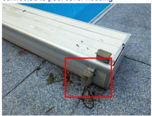
**39:** The electrical wires in the pump area were not protected. Recommend putting them into a protective conduit.
